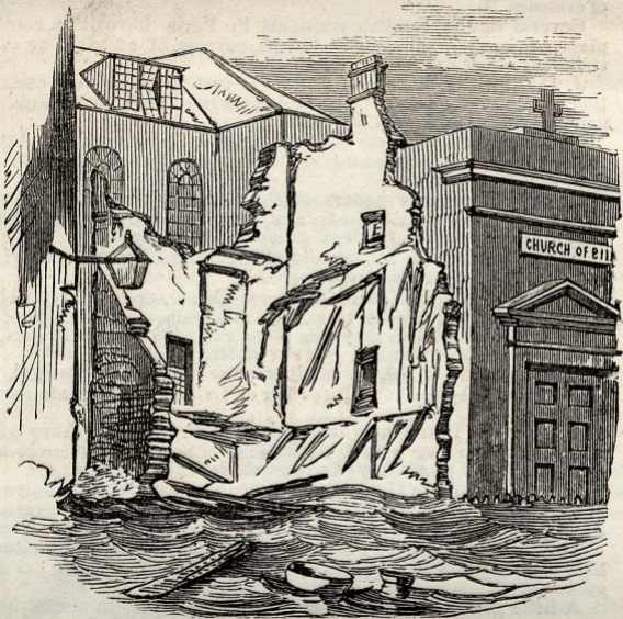
REMAINS OF FALLEN HOUSE IN FISHAMBLE-LANE, CORK.
