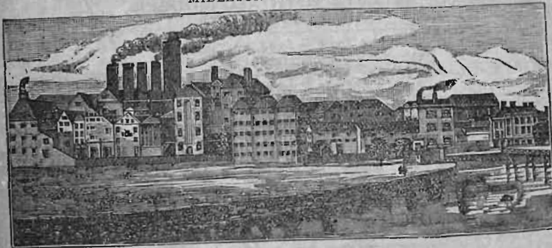
NORTH MALL DISTILLERY.
