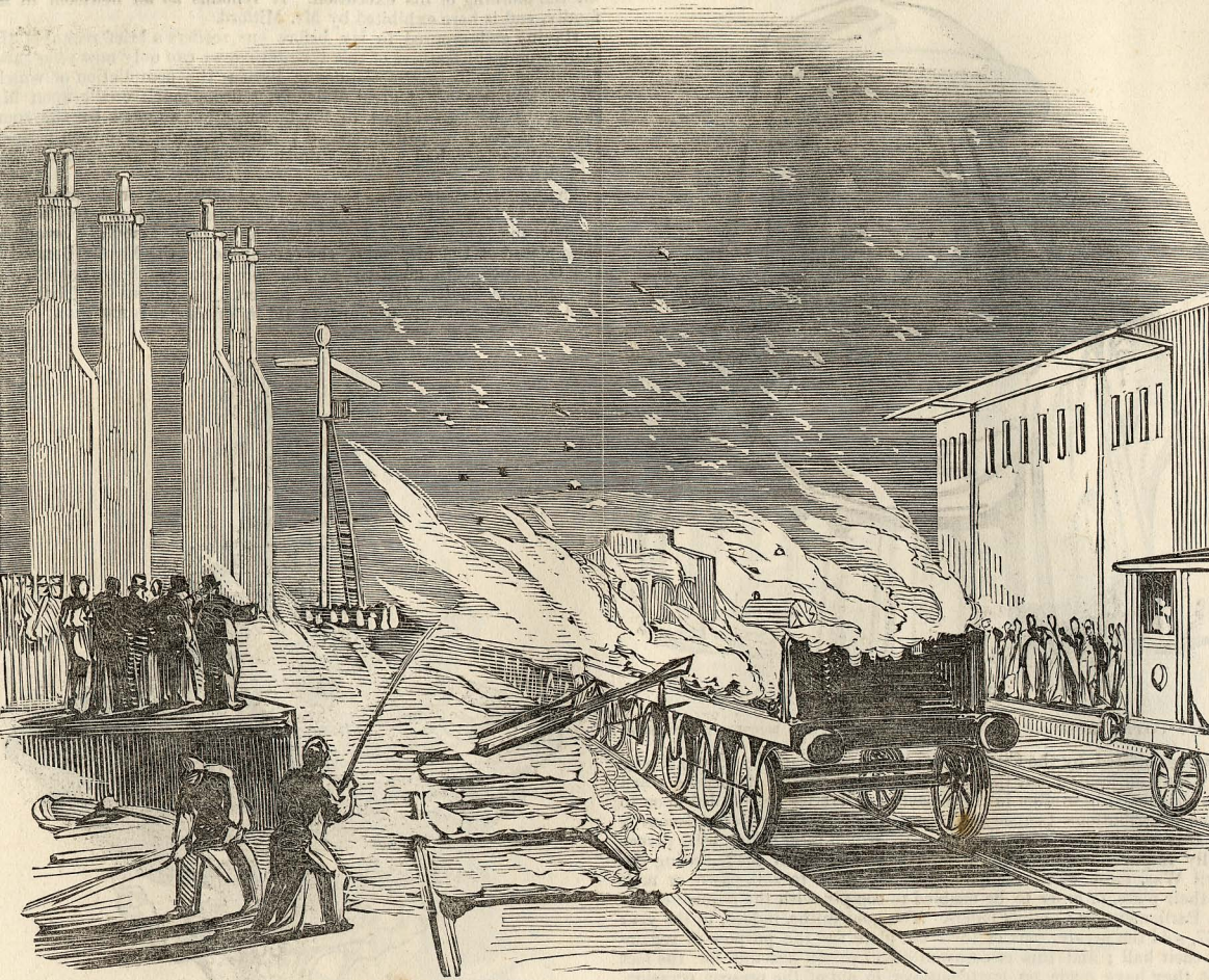
GREAT FIRE AT THE SOUTHERN AND WESTERN RAILWAY STATION, CORK.
