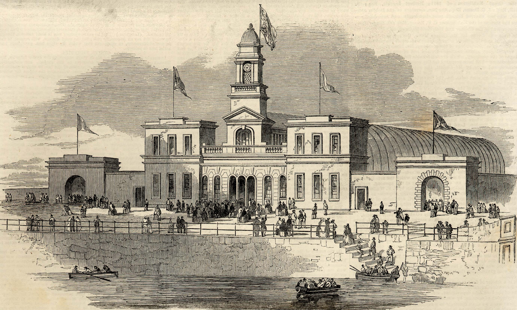
BUILDING AT CORK FOR THE NATIONAL EXHIBITION OF THE ARTS, MANUFACTURES, AND MATERIALS OF IRELAND—(SEE NEXT PAGE.)
